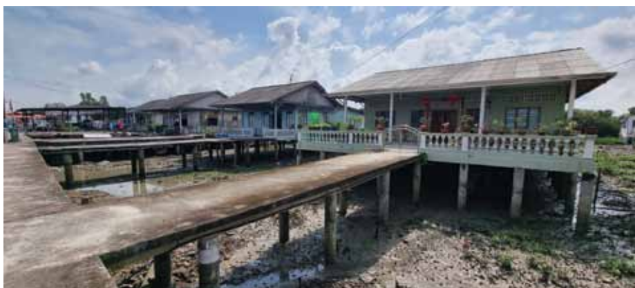
Kukup boasts entire villages suspended over the sea on concrete stilts and platforms.
