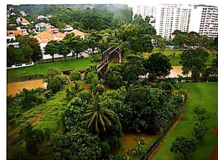
Jurong Line crossing Sengkang Pandan.
